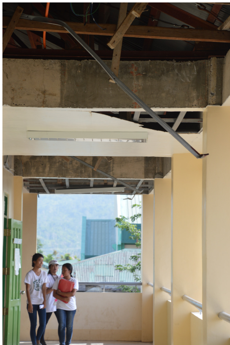
DANGER ZONE. Senior high school students from Catanduanes National High School fear that damaged ceilings and roof brought by Typhoon Nina's wrath might trigger serious dangers – this time, jeopardizing lives. GVALLEDOR
